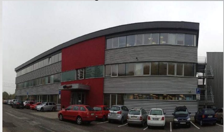
Picture n. 1 : Hall „C“ / Administration building
