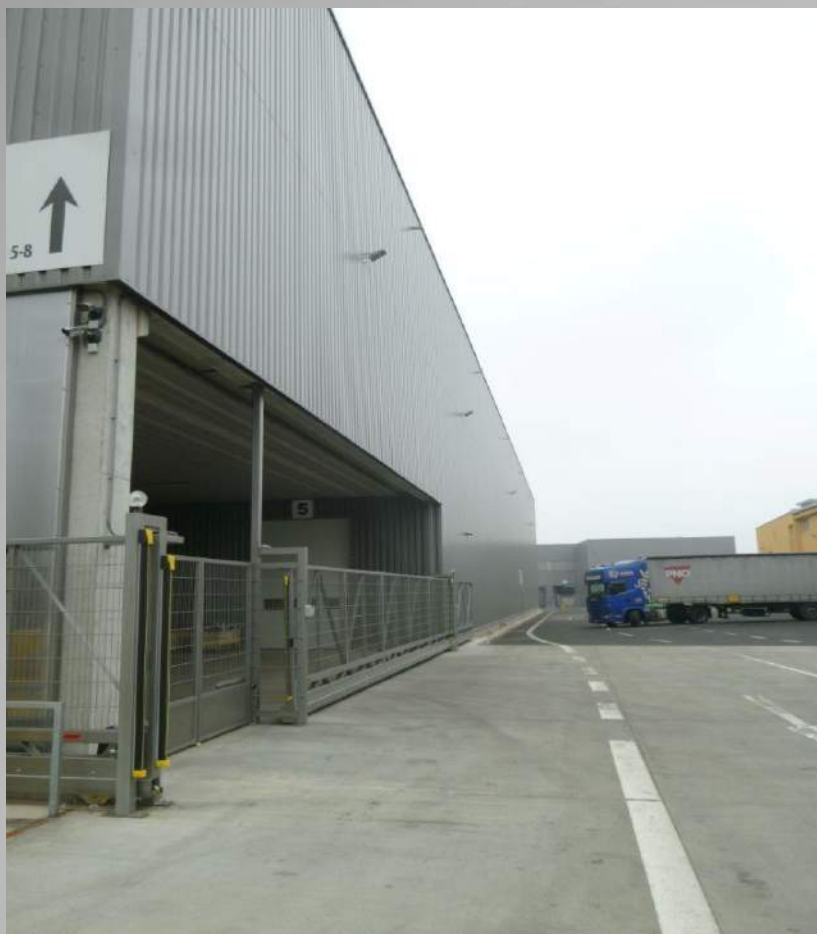
Picture n. 5: Exterior or warehouse spaces of Halls „A“ and „B“
