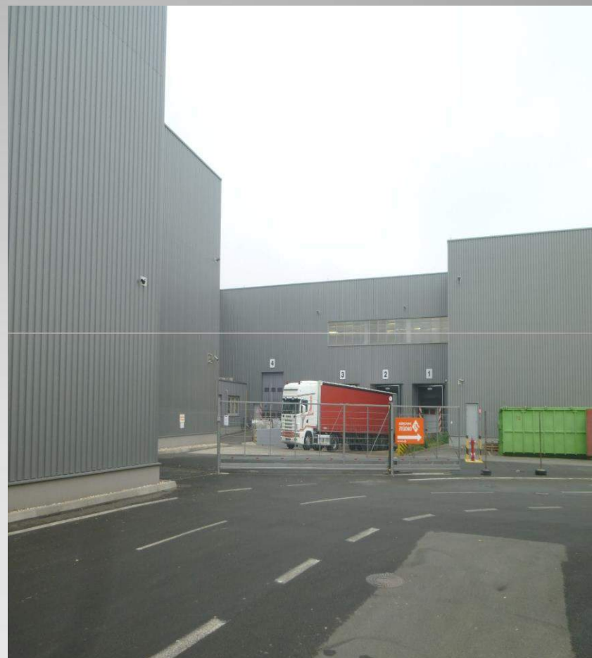
Picture n. 6: Exterior of warehouse spaces of Halls „A“ and „B“
